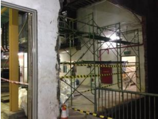
Demolishing wall for unloading
