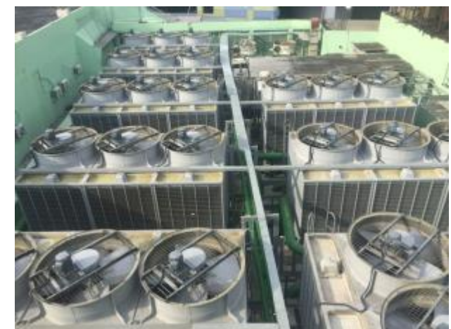
Cooling Towers after replacement
