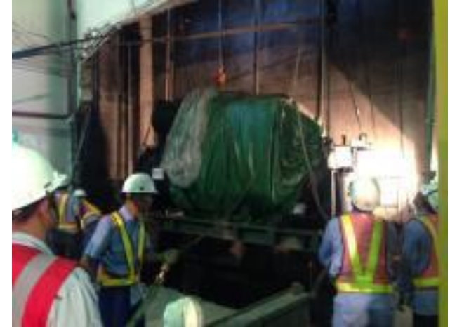
Lifting Chiller from unloading shaft
