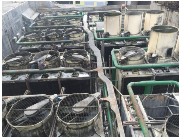
Cooling Towers before replacement
