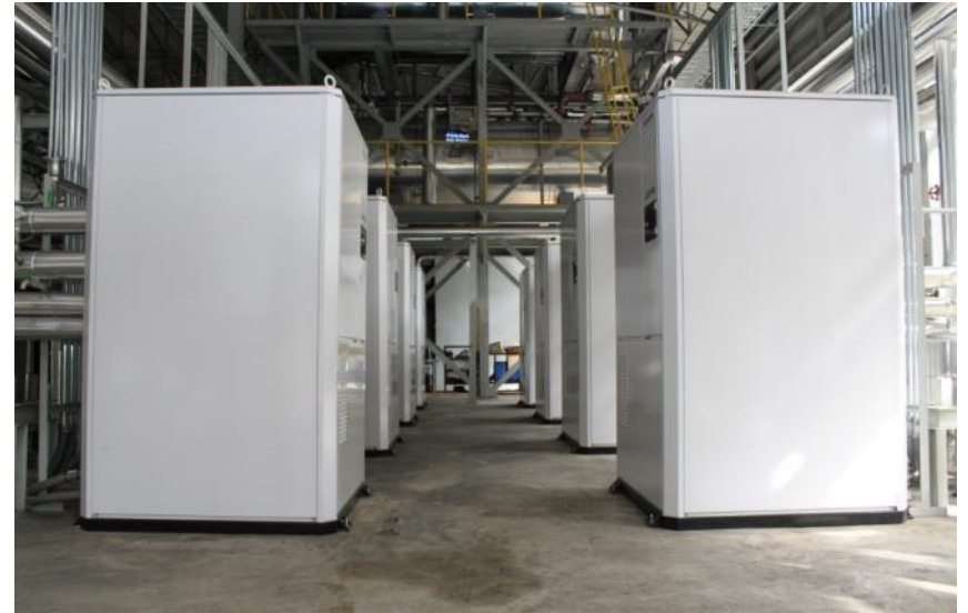
Heat Recovery Heat Pump Systems
