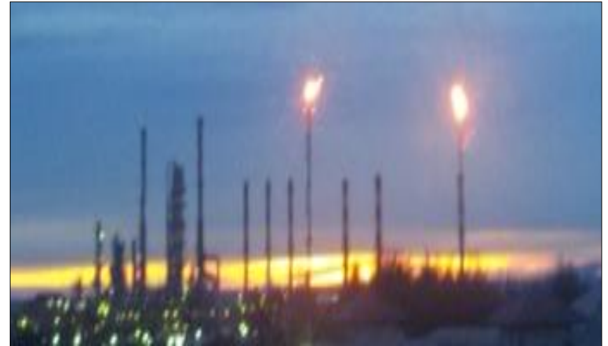
Refinery Unit V (View from Blue Sky Hotel )
