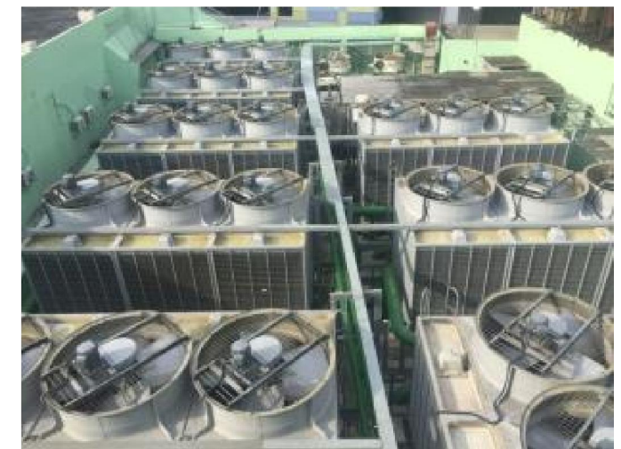
Cooling Towers after replacement
