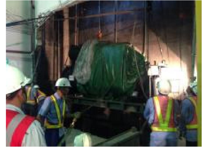
Lifting Chiller from unloading shaft
