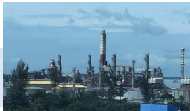
Refinery Unit V In Balikpapan, East Kalimantan
