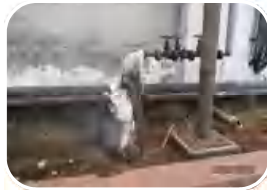
main pipe condense extraction
