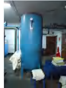
Figure 6-11 Air receiver in GKL
