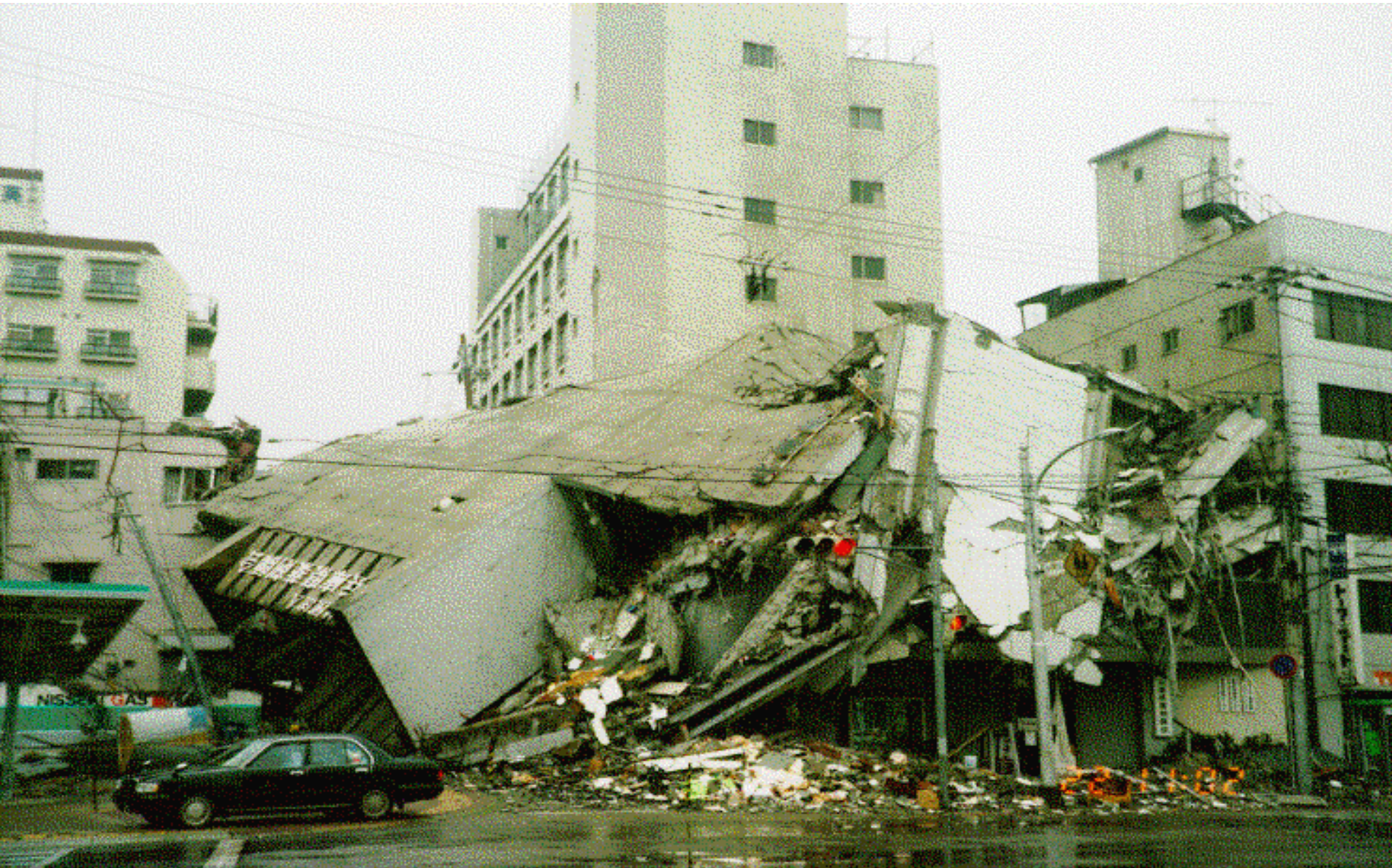
Kobe damaged by the Great Hanshin-Awaji Earthquake (1995) 阪神・淡路大震災（神戸）
