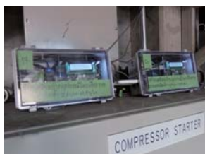
19-1 Compressor Monitoring Devices Utilizing IoT
