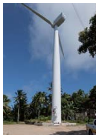
No.17-3 300kW Wind turbine generators with typhoon resistant system
