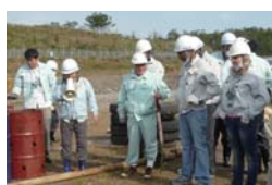
Practical exercise for constructing the sanitary landfill (in course B)
