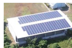
No.12: Solar PV System for Schools Project (Palau)
